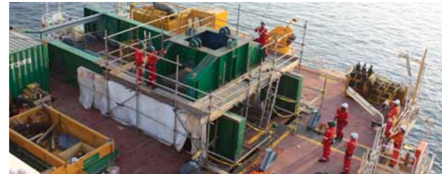
Preparations for the offshore Stream-1 flare tip replacement
