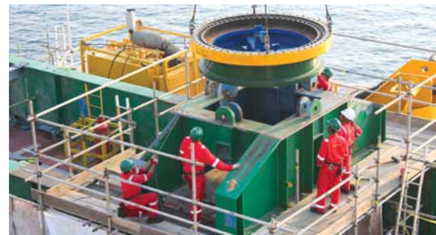
The AGR-1 gas cooler tube bundle pulling operation
