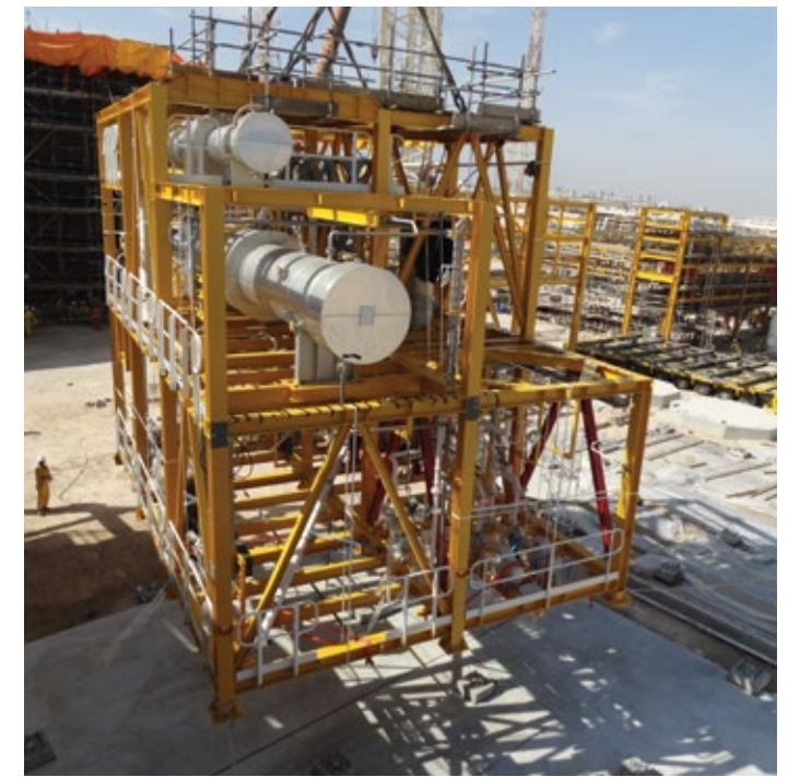
Delivery of Evaporator Package
