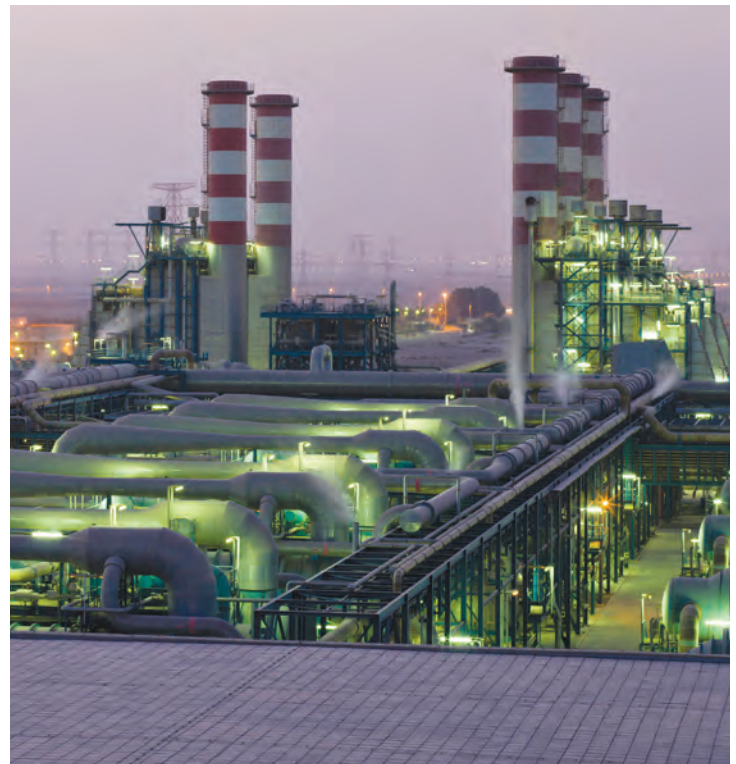
Taweelah A1 Power Plant
