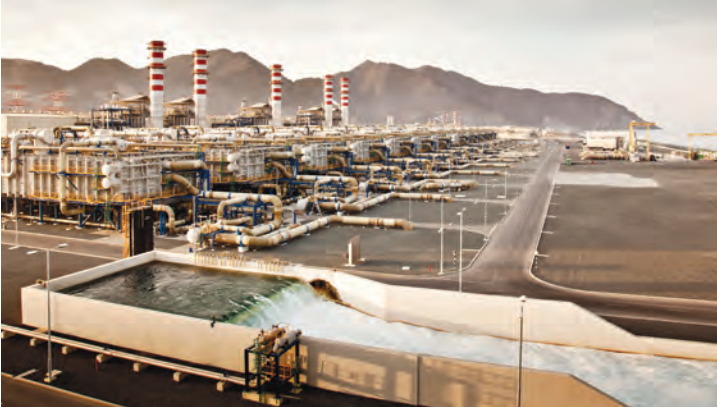
Fujairah F2 Power Plant
