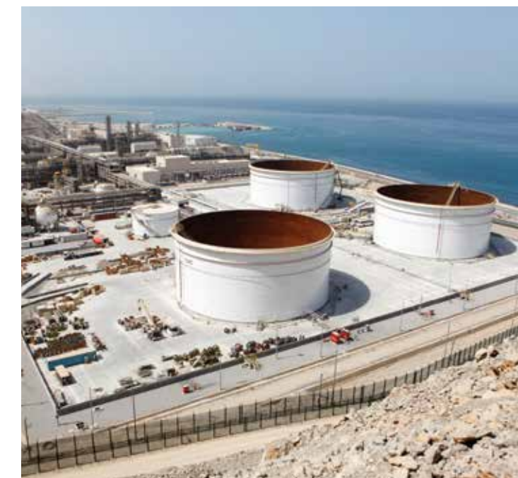
The Musandam Gas Plant in Oman
