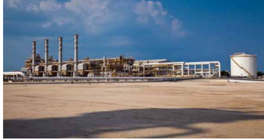
Our Gas Processing Plant at Ras Laffan
